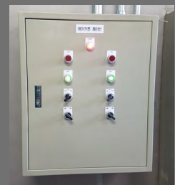
Control panel production
