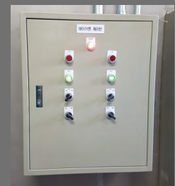
Control panel production
